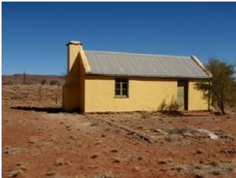
Namatjira's house, Hermansburg
